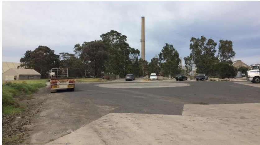
Figure 3-2: Existing concrete hardstand
