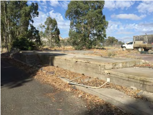
Plate 4: Raised slab on the eastern side of the former Mill buildings
