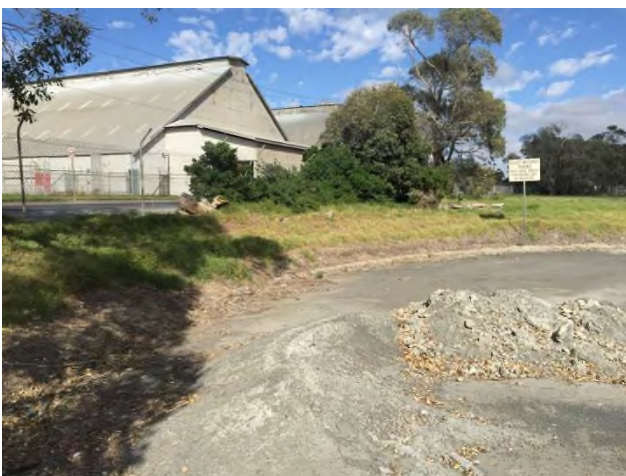
Plate 8: Southern end of the carpark road showing cutting below level of Walchs Road
