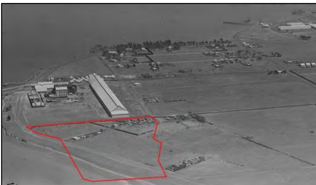
Plate 1. Historical photo (1938) of the study area, showing the original Corio Bay shoreline: photo direction: south
